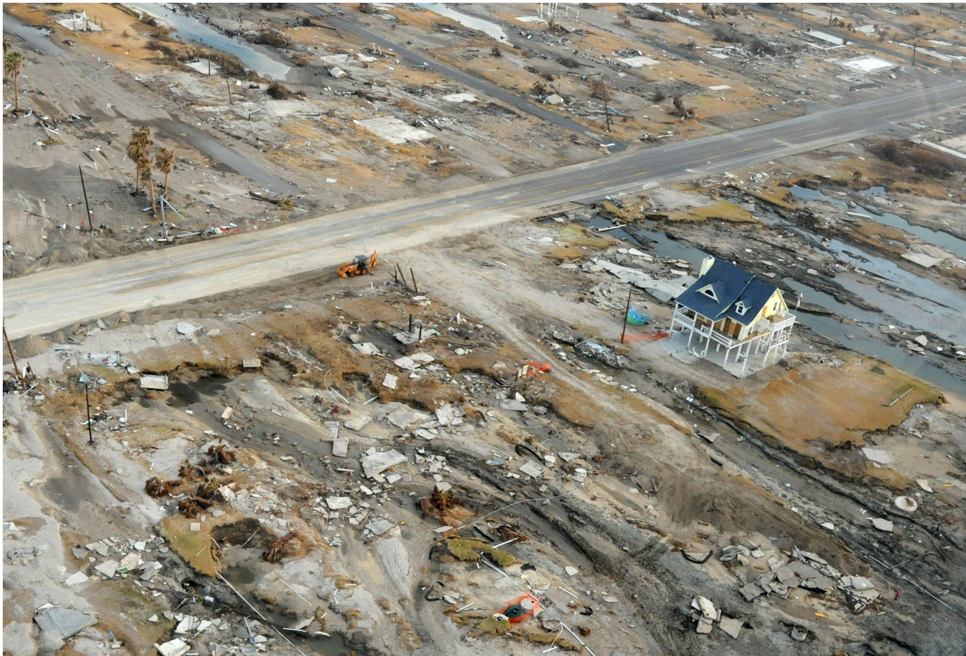
A home in Gilchrist, Texas, designed to resist flood waters survived Hurricane Ike in 2008. Credits: FEMA/Joselyne Augustino
